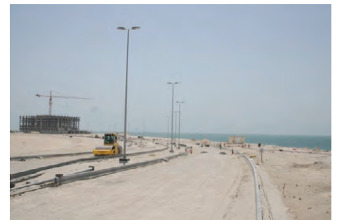
Work in progress on the distributor road ahead of asphaltting
