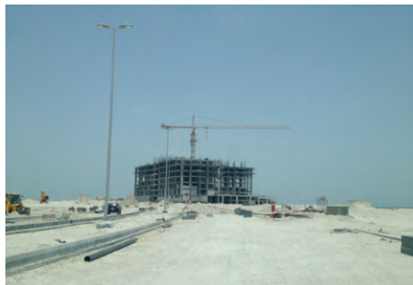
Construction progress at The Treasure
