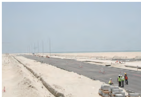
A view of arterial road works, with street lighting being placed
