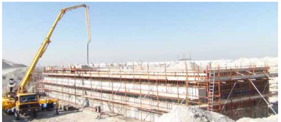
Distributor bridge side structure
