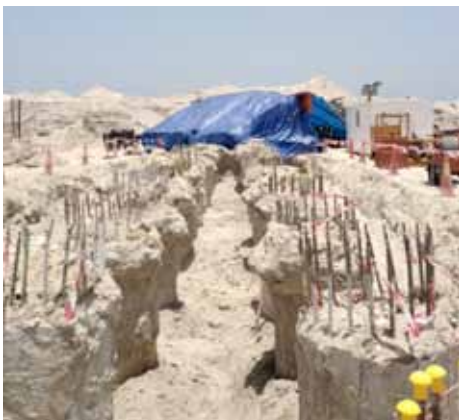
Bridge piling works
